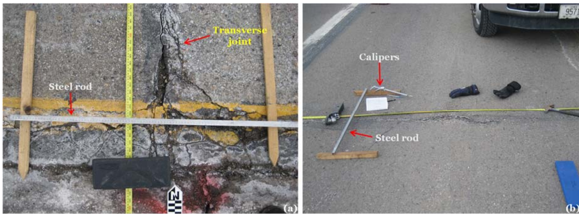
Figure 4.3. Measuring vertical heaves at transvers joint locations.
